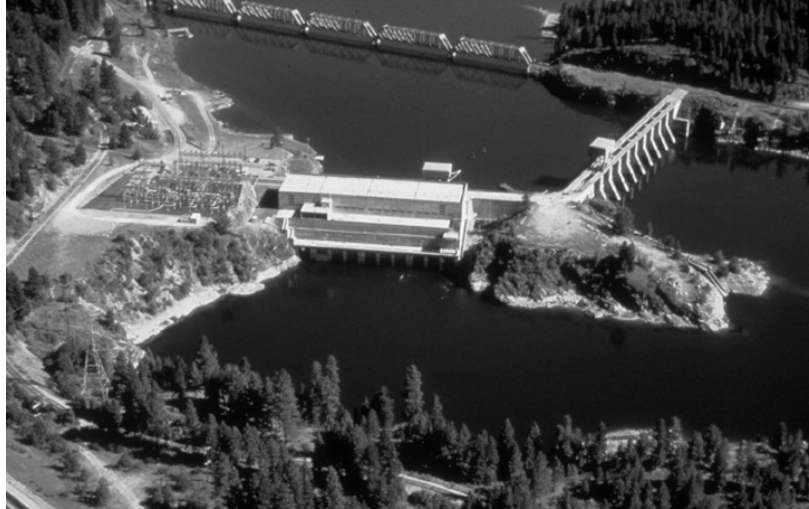
Albeni Falls Dam. U.S. Army Corps of Engineers.
